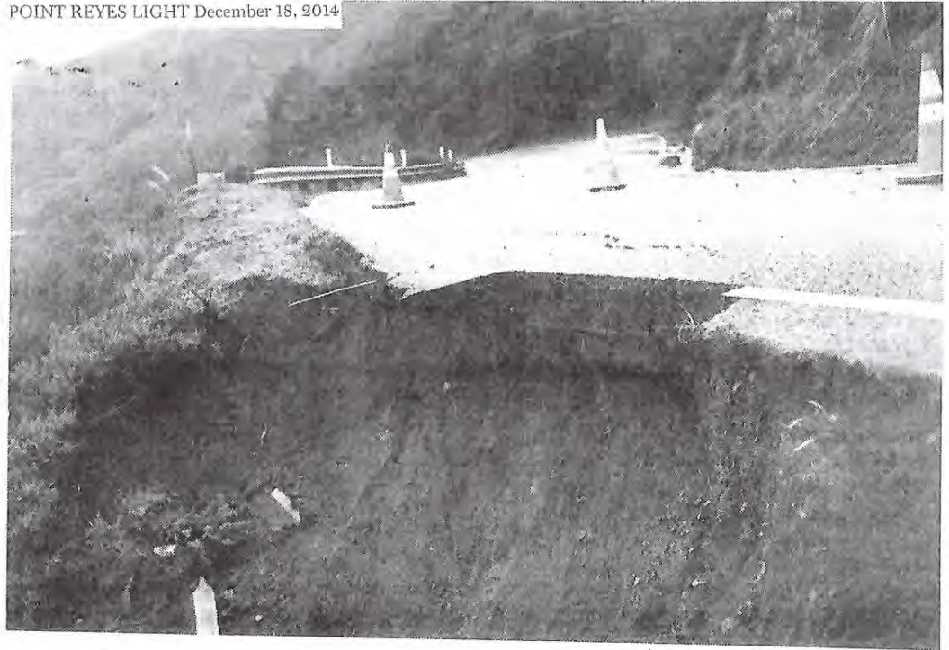
MUIR BEACH: Thursday's rains washed away soil beneath a portion of road on Highway 1 between Panoramic Highway and Muir Woods Road, causing the roadway to crumble. Caltrans estimates that the affected stretch will be closed until March.
